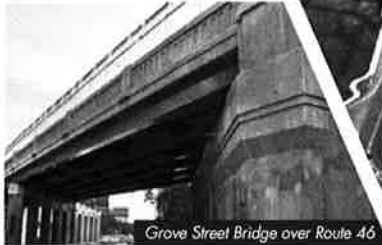
Grove Street Bridge over Route 46
