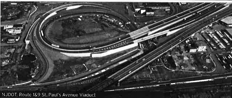
NJDOT, Route 1&9 St. Paul's Avenue Viaduct
