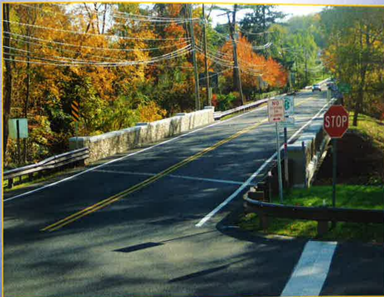
U.S. Route 202 over Passaic River Bridge Replacement
